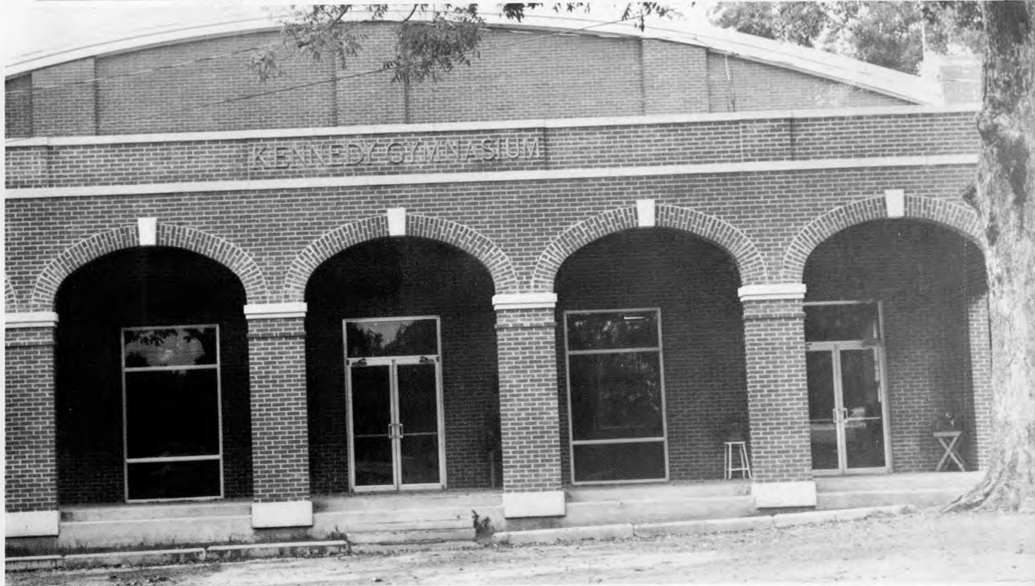
Kennedy Gymnasium- a new lobby
